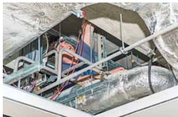
The cables for the rebuilding of the fire protection systems are being relaid in the intermediate ceilings.
