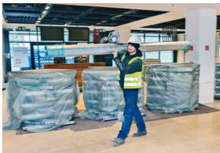
Ventilation ducts are being laid to provide the right ventilation.
