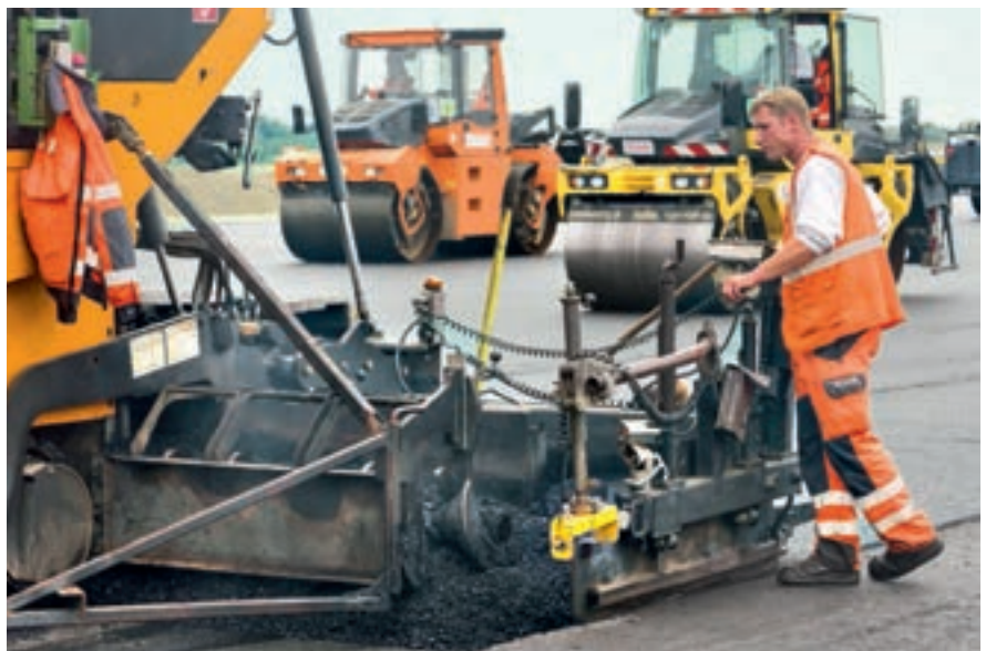
Up to 200 construction workers were employed on the North Runway between May and the end of September 2015. Using about 50 units of heavy equipment such as milling machines and asphalt finishers, the workers removed the two old upper asphalt layers and laid new asphalt on around 220,000 square metres.
