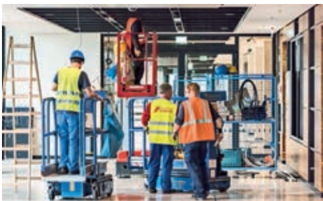
Schulzendorfer Elektro is installing the cables for smoke windows in the Main Pier.
