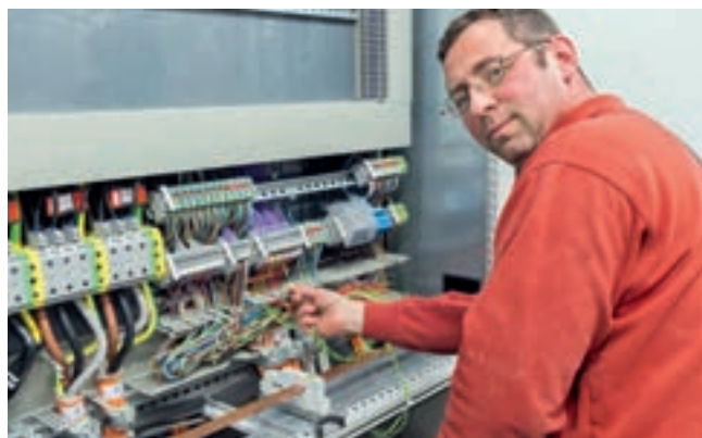
Low-voltage power lines are connected for a segment of the GSPLCs.
