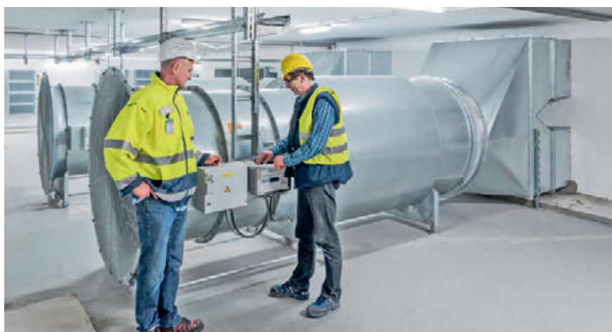
Ducts for the replenishment air in the delivery bay south
