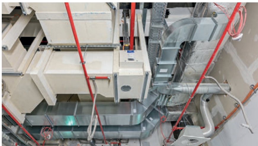
Retrofitted smoke extraction flues and sprinklers, before the intermediate ceiling is drawn in
